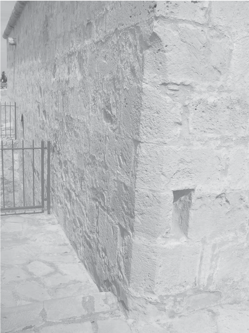
Fig. 50: Limassol Castle, roof level, chambers above the réduit , detail of chamfer in southeast angle [M. Olympios].
